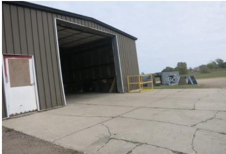
CIVIC CENTER - COLD STORAGE
